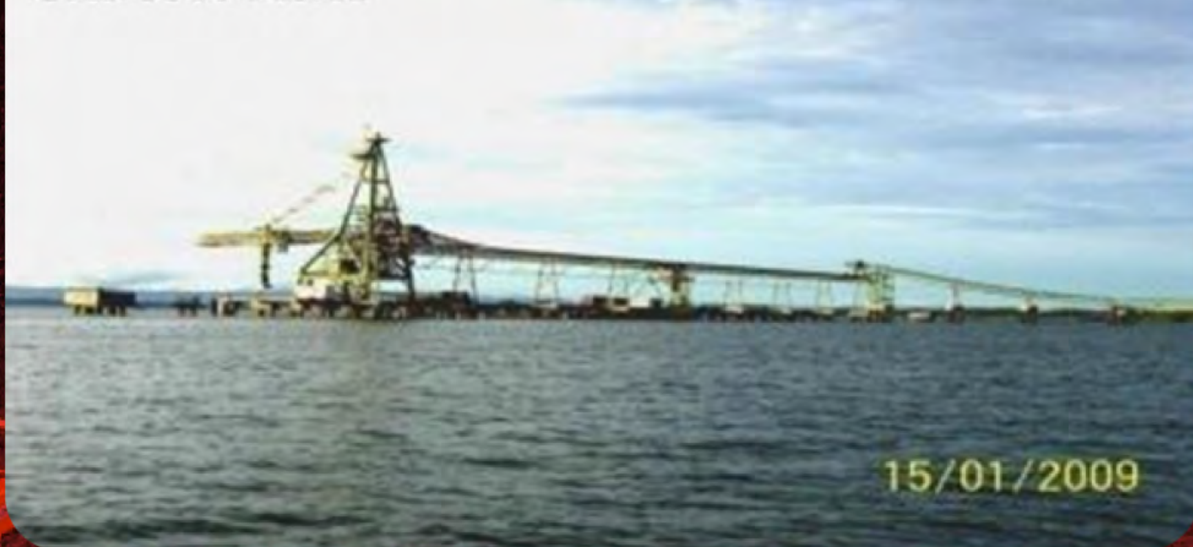
SHIPLOADER & WHARF CONVEYOR CAP 3500 M3/H
